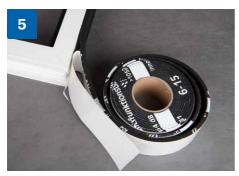
> Mount Ampacoll Komprimax flush with the inside of the frame. Lav without tension.
