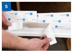
> Where the sealing foils meet, make sure that the ends overlap and that the connection is airtight, windtight and impermeable to driving rain.
