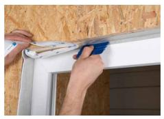
> Stick the first side of the window to the wall. To do this, remove the liner step by step, align the adhesive tape and apply it tension-free (relief loop). Rub or press on well.
