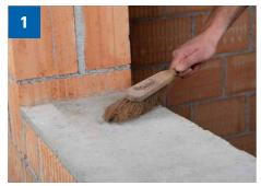
> Surfaces must be dry, frost-free, loadbearing and free of dust, separating agents and grease. Clean surfaces thoroughly and check load-bearing capacity.
