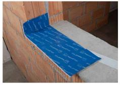
> Mark the position in the reveal. Cut Ampacoll® Sillskin to length allowing for lateral overlap, then firmly press on the adhesive tape. Side overlap: DE  $\geq$  10 cm; AT  $\geq$  6 cm. Note: The example does not show an inclination for the window sill base. The inclination can be part of the wall element or can be created by installing a gradient wedge.
