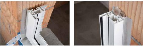
> Stick Ampacoll® Fenax DS for alternating bonding to the inside and outside of the window frame, then press on well. Create corner loops: approx. 1.5 × joint width. Insulate joints ensuring there are no cavities. Create relief loops.
