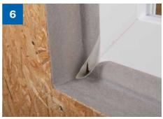
> Tip: Circumferential installation of Ampacoll® Fenax after window installation (without incision and in a single pass). The corner can be made without cutting by creating an inverted pleat.
