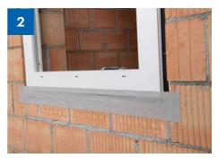
> Start at the bottom, then the sides, then the top (water flow)
