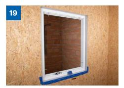
> Stick the second side of the frame to the wall. To do this, remove the liner step by step, align the adhesive tape and apply it tension-free (relief loop). Rub or press on well.
