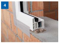
> Insulate joints ensuring there are no cavities. Material as specified by the planner.
