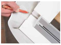
> Any corners and grooves in the profiles must be airtight or windtight and protected against driving rain. For this reason, the window connecting tape for this window was placed further inwards.
