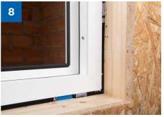
> When using support blocks, cut out the multifunctional tapes. The cut-out must be narrower than the width of the support block (airtightness).
