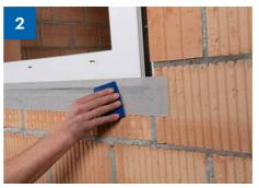
> Rub the adhesive tapes on well using the Ampacoll® Pressly press-on aid.
