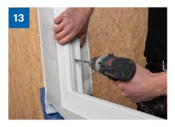
> Initial situation: Built-in window frame with prefabricated adhesive tape skirt. Decide whether to start the installation on the inside or outside depending on the local conditions or the specifications of the planner (consider weather conditions and construction progress).
