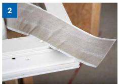
> Used window connecting tape Ampacoll® Fenax 30/45 DS (double sided, adhesive surface on front 20 mm).
