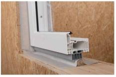
> Stick Ampacoll® Fenax DS for alternating bonding to the inside and outside of the window frame, then press on well. Create corner loops: approx. 1.5 × joint width. Insulate joints ensuring there are no cavities. Left: without window connection profile (FBA). Right: with FBA. Note: Observe the design of the window sill base, see pages 17-19 second sealing layer / window sill base.
