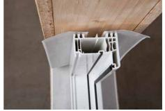
**Example:** On the left, the two prefabricated Fenax skirts. On the right, central installation in wooden frame wall. Insulate joints ensuring there are no cavities. Apply the Ampacoll® Fenax adhesive tapes tension-free or with a relief loop.
